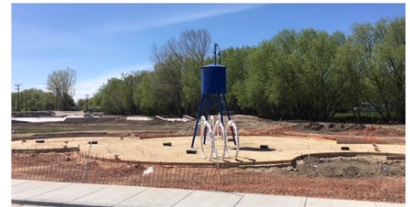
Construction progress as of 4/23/18
