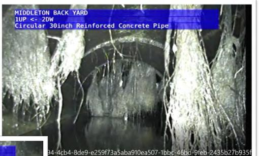
Video inspection of the drain revealed significant root blockages. Behind the blockages, significant rocks and sediment build up further restricted flows.
