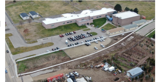
Sidewalk Constructed with Child Pedestrian Safety Funds
