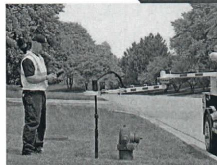
ERV-750 extended reach valve exerciser allows valve operation from the road, removing the need to pull onto the grass
