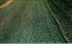
stages will resemble a chicken wire or alligator pattern. Some common causes of fatigue cracking are loss of base support due to poor drainage, increased heavy traffic loading, inadequate structural design, or
