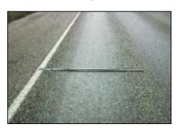
continue to densify under traffic loads. Subgrade rutting occurs when the subgrade fails due to settlement or lateral movement. In this case, the pavement settles into the subgrade ruts causing the surface depression in the wheel path. The method of repair depends on the type of rutting. Severe pavement rutting should be repaired by a mill and overlay. Subgrade rutting can only be repaired by replacing the entire pavement and failed base.
