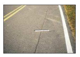
However, if not addressed early they will continue to ravel, widen, develop into multiple cracks, and allow moisture to penetrate and weaken the base and sub-base.
