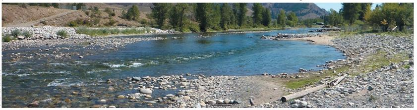
**Solution B:** Low-profile barbs can improve channel complexity. The picture above is taken between two low-profile barbs constructed of logs with native bed material backfill. The barbs were designed to overtop at bankfull flow. Note the slow water between the barbs and the well-defined thalweg.
