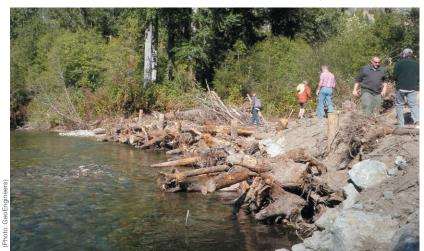
**Solution:** Root wads can be an alternative to rip-rap and other bank structures. When coupled with riparian plantings and lowering of floodplain surfaces, the floodplain can be reconnected to the channel and habitat value increased for many species.
