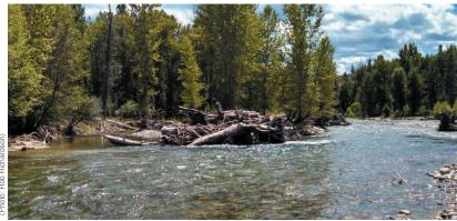
**Solution A:** Well engineered logjams and boulders placed in the channel can create split flows. Point bars form behind and back bar side channels around them and are active at a wide range of flows.
