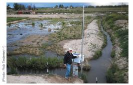
North Alkali Drain Water Quality Improvement Pilot Project, Parma. Implemented in 2014 by Integrated Watershed Solutions, this project tests whether a sedimentation basin in combination with constructed wetlands can remove significant quantities of sediment and phosphorus from irrigation return waters. Initial results show effective removal of both pollutants.
