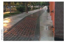
Green Stormwater Infrastructure, permeable pavers, Boise. Installed in 2015 by the Ada County Highway District (ACHD), the pavers help eliminate standing water through infiltration and clean rain and snow melt; they are both cost-effective and aesthetically pleasing.
