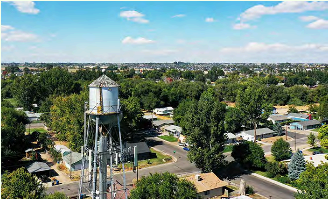
Middleton Water Tower. Source: Mike Brown Group
