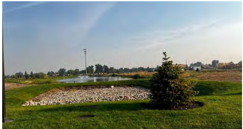
Example of retention pond for stormwater management in Middleton
