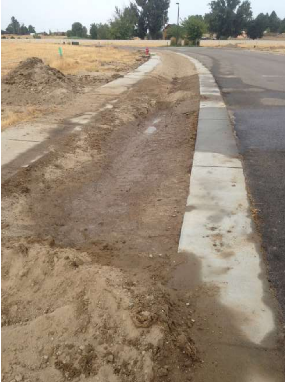
Photo 2 - This older photo (circa 2014) from Powder River 2 subdivision showing construction photo of the swale just before acceptance; Example where sand strip is missing or is covered by soil, which likely lowers rate of water infiltration
