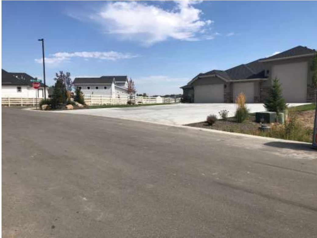
Photo 4 - Bard Street residence constructed around 2020; example of home with no swale showing the “disconnect” between stormwater design/building permit phases and final construction.
