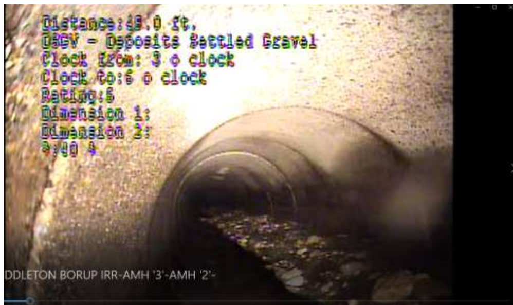
Photo A2 – Gravel in pipeline after cleaning
