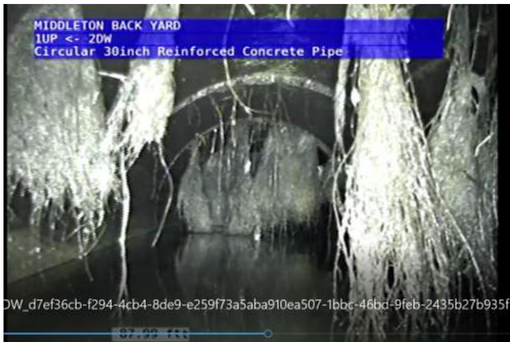
Photo A3 – Roots in pipeline after cleaning
