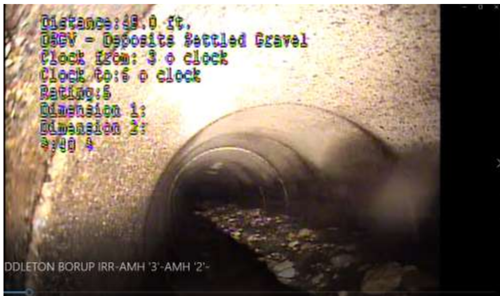
Photo A2 – Gravel in pipeline after cleaning
