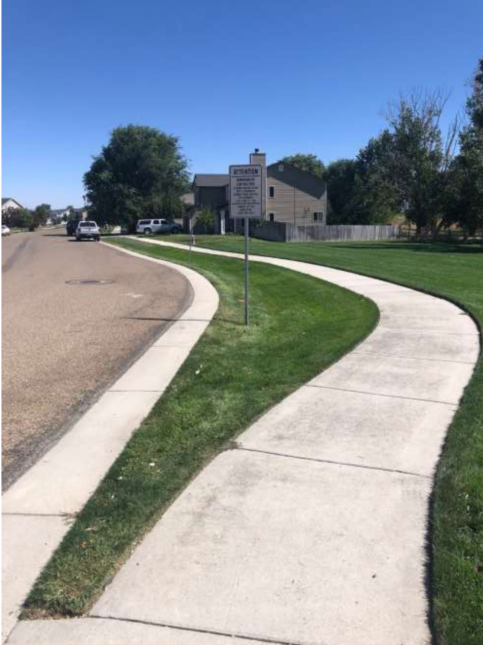
Photo 3 - Swale in Condor in Falcon Valley 2 constructed in ~2010; post occupancy and with ongoing maintenance swale appears to functioning; example showing of older BMP without sand strip; infiltration rate may be reduced
