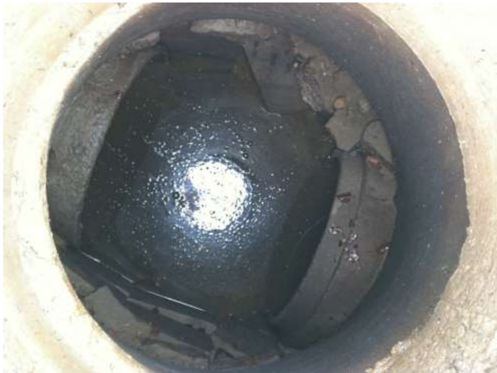
Photo A1 Manhole showing inflow/outflow connections
