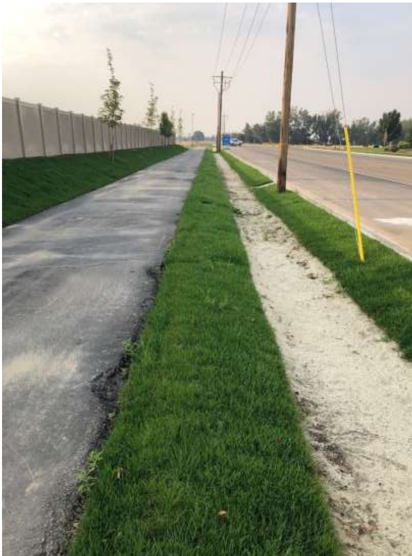
Photo 1 - recent (Aug 2022) finished swale showing sand strip that allows water to infiltrate
